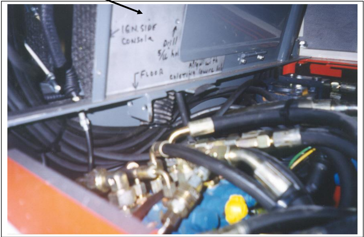
Front mounting hole template in place
